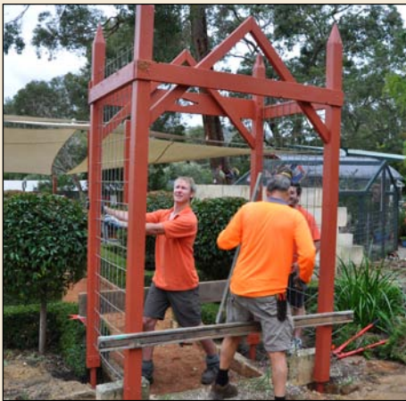
Alec, Graeme and David installing the gate
